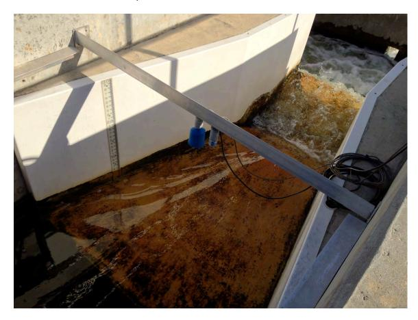
Standard Openchannelflow staff gauges are marked in centimeters on one side and feet / tenths / hundredths of a foot on the other. Custom gauges are also available, usually graduated in flow on one side and level on the other.
