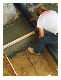
9) In determining the elevation of the concrete slab, refer to the manhole design drawings provided by Openchannelflow.com in the equipment submittal, making sure to allow for the 1/2 inch [1.27 cm] thick foam pad (provided with the manhole) that fits between the manhole barrel and the concrete slab.
