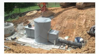
17) For flow monitoring and grinder manholes, check that the interior structure (flume / weir / grinder channel) is level, adjusting as necessary. For flumes verify the level at the inlet floor of the flume. For weirs verify the level at the face of the weir. Do not level flume flow monitoring manholes by leveling the top of the flume – level the inlet floor of the flume. Minor level variations should not affect diversion / flow control, energy absorbing, or storm water manholes.
