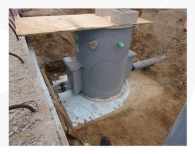
10) Where buoyant forces are very high due to a high water table, the flume / pipe stubs may be encased with reinforcing concrete – poured in 6 inch [15.24 cm] lifts – up to the top of the flume.
