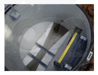
30) The void space may be on either side of the structure in the manhole and extended under the structure.
